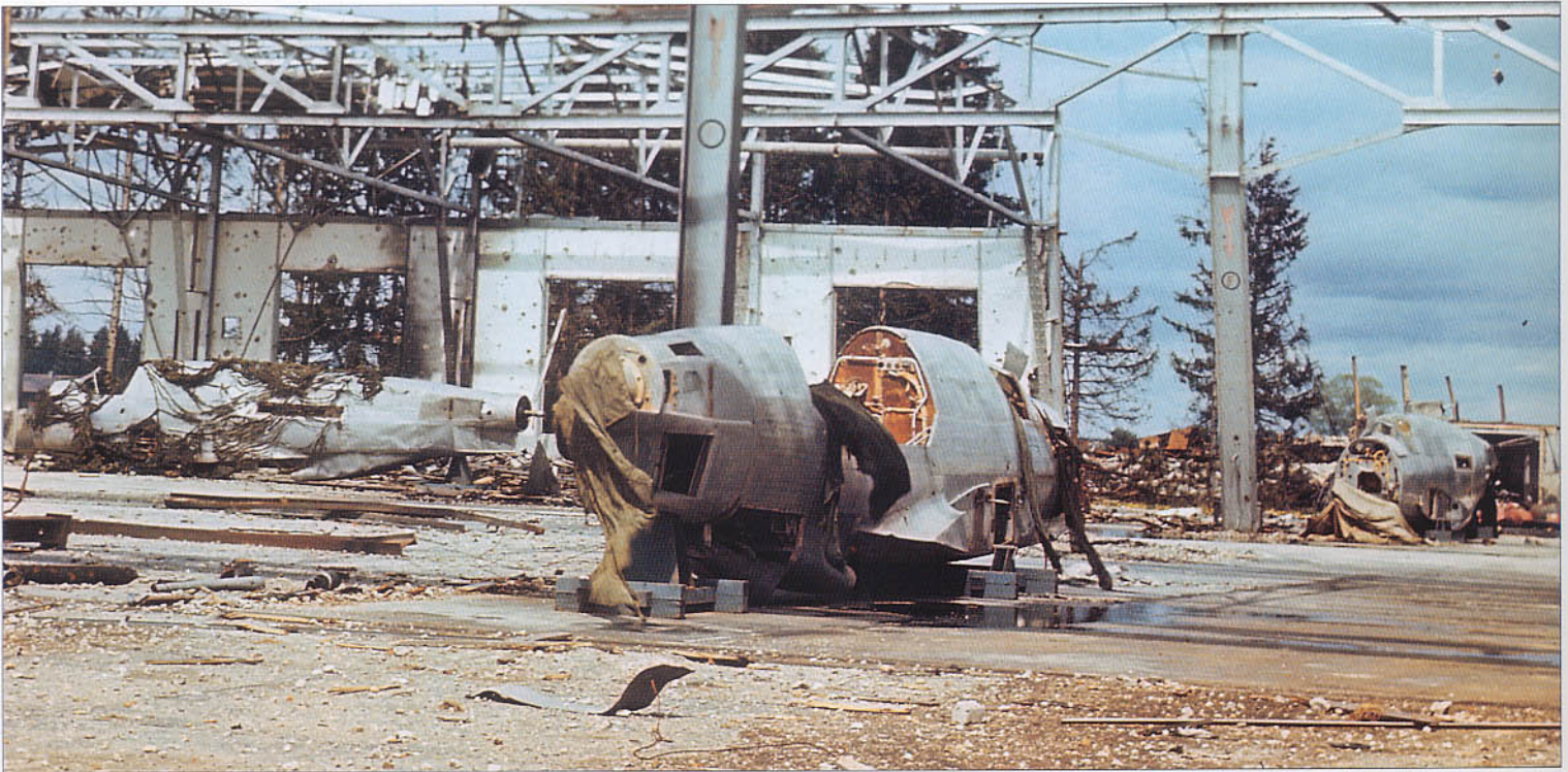
Above: One of several B-series fuselages found partially assembled at Dornier's Oberpfaffenhofen facility. Judging from the condition of hangar, these hulks were abandoned after an Allied bombing attack.
